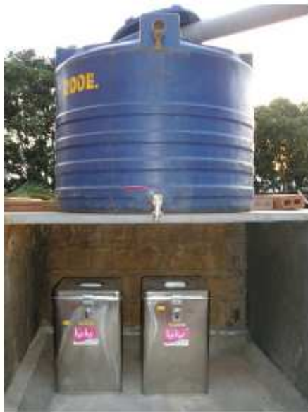
Waste composting in two tin drums 'Tippy tap' for washing with minimum water below the rain water collection drum
