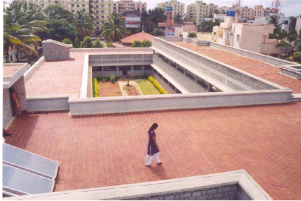
Figure 4: Every rooftop needs to be kept clean to act as a good catchment for rainwater
