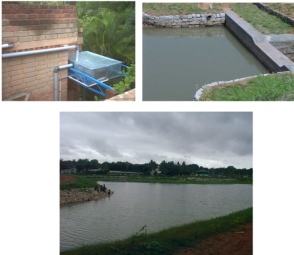
Fig 7 : Storage devices are many from a roof tank to a lake
