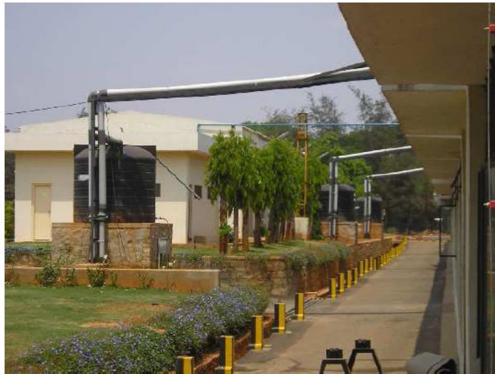
Fig 10: Rain barrels at work harvesting rain in a factory
