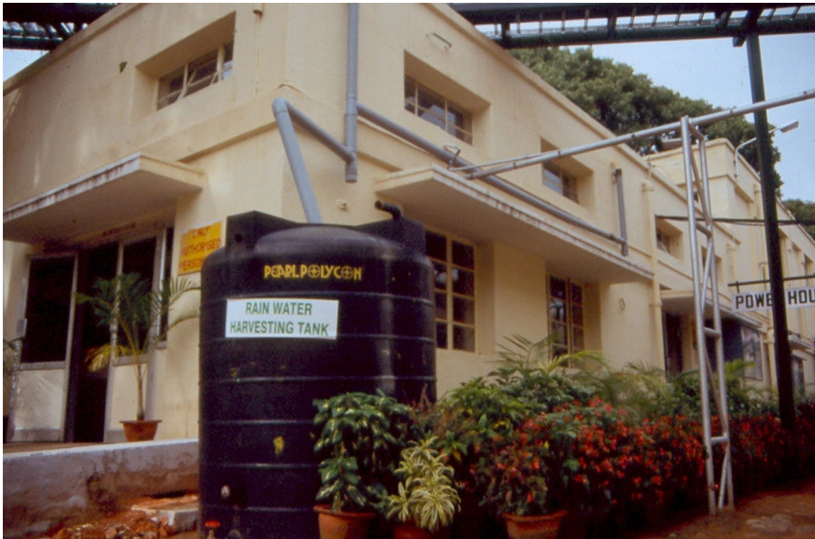
Rainwater Harvesting for an industry to a Rain Barrel
