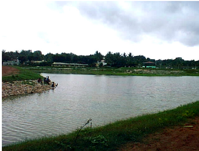
Fig 4 NARASIPURA-1rainwater harvesting for groundwater recharge
